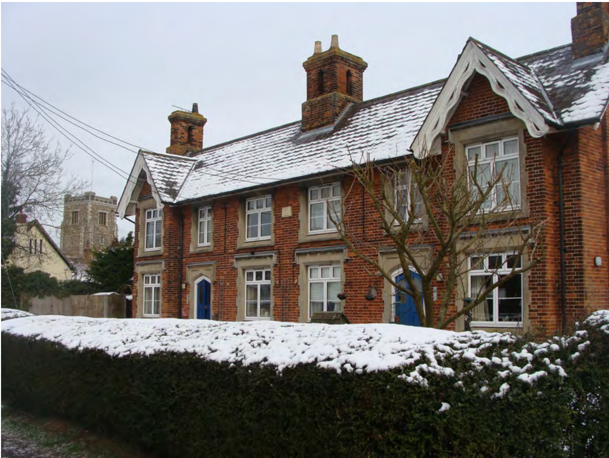
Picture 1.12 Former late 19th century almshouses with several distinctive architectural features worthy of preservation, possibly by Article 4 Direction subject to further consideration and notification
