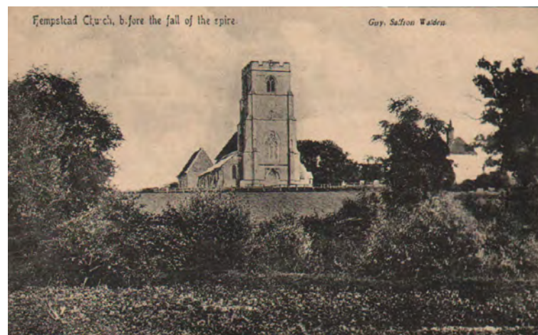
Picture 1.2 Hempstead church "before the fall of the spire" from a postcard published by Guy of Saffron Walden. The west tower (15th century) collapsed in 1882 and was rebuilt to nave height in 1933-4 in memory of William Harvey (1578-1657). The tower was completed to its present height in 1959-60. (Reproduced courtesy of Saffron Walden Museum)
